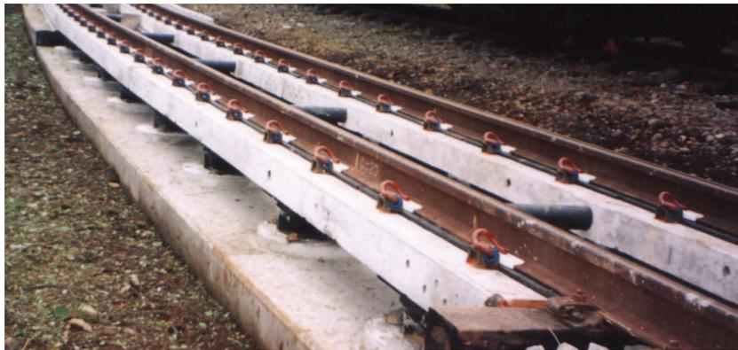
Figure 1: FLT test installation at the RTRI (courtesy H. Wakui).
